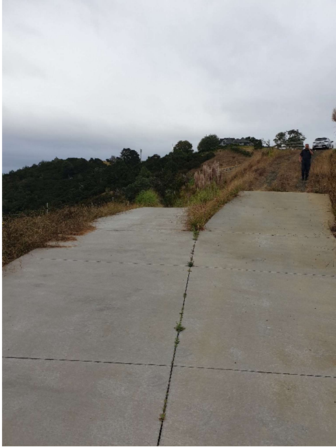
JUNCTION ON PRIVATE ROAD
